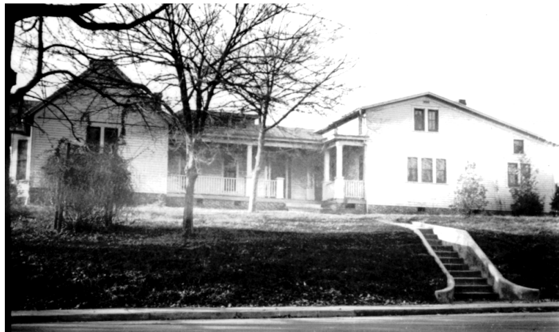
The Grey House / Kilgore House home of Kate and Fred Ganter Across the street from 321 Washington Street
